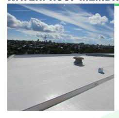
Viking Silcoat is a liquid membrane system that can be applied to virtually **any existing roof surface** to extend its life.
